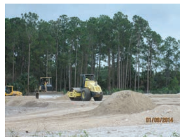
But Terracina Grand II is being built.
